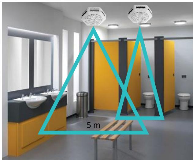
Sensor covers ~2 – 2.5 meter radius zone. Best sensor mounting height is up to 3 – 3.5 meters.
